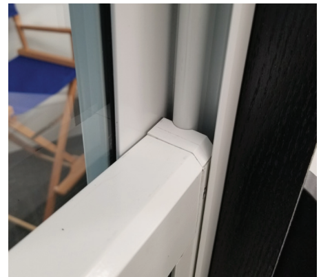
Sash cover guide (small for eze lift/large for ultra)
